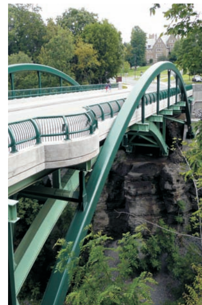
Bridge with catenary-shaped support (Cornell University, Ithaca, NY).
