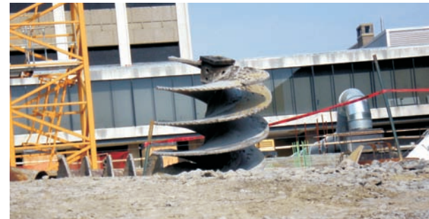
Double-helicoid auger on a construction site, Cornell University.
