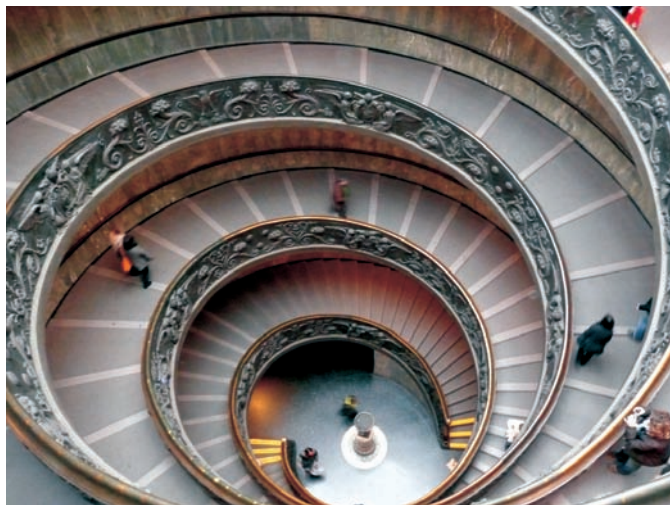
Double helicoid with the center removed: exit stairway in the Vatican Museums.
